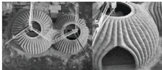
Figure 4:3d printed units using earthen walls with integrated voids for electrical and plumbing connections
